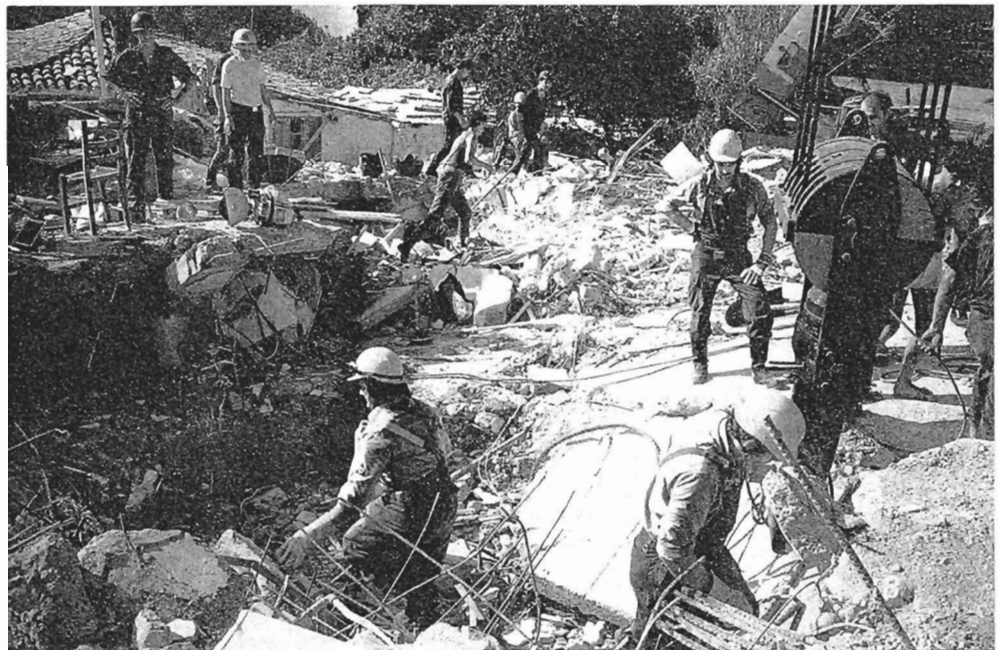
Right: Search and rescue operation on a collapsed six storey reinforced concrete apartment building (Kalamata earthquake, Greece, 1986)
