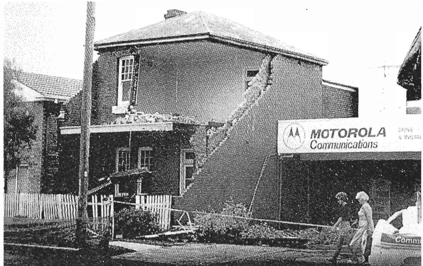
Right: Front and side collapse in modern unreinforced brick masonry, two storey dwelling in the 1989 m_b = 5.4 Newcastle earthquake, Australia
