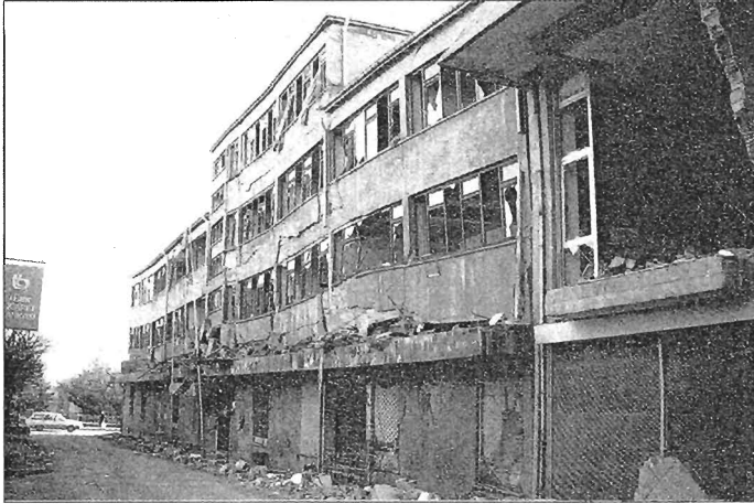
Top left: Example of collapse starting from the ground floor (Kalamata, 1986)
