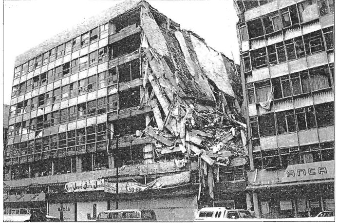
Top Right: Example of top-down collapse. This building was originally 11 stories high. The bottom 3 floors and part of the 4th floor are still standing (Mexico City, 1985)
